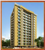
Tower Four - exterior view, front facing.
